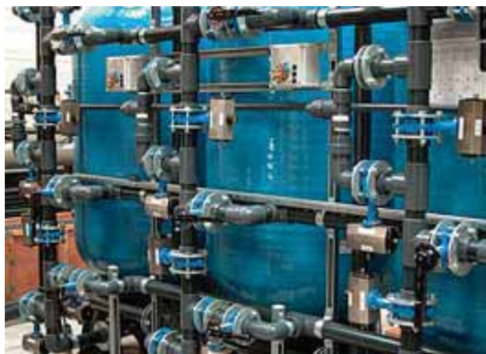
Picture supplied courtesy of Sterling Hydrotec.
